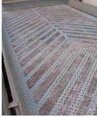
Ramp with Belzona 1821 chevrons
