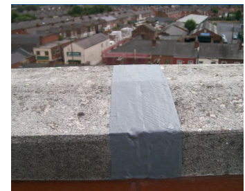
Parapet walls & coping stone joints
